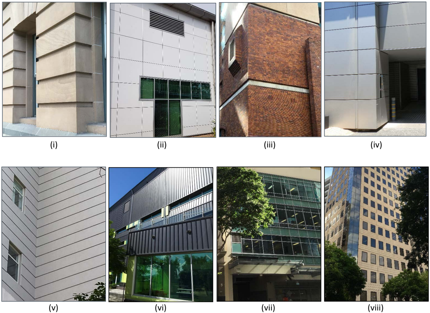
Figure 5: Queensland buildings with various types of external wall materials/cladding
