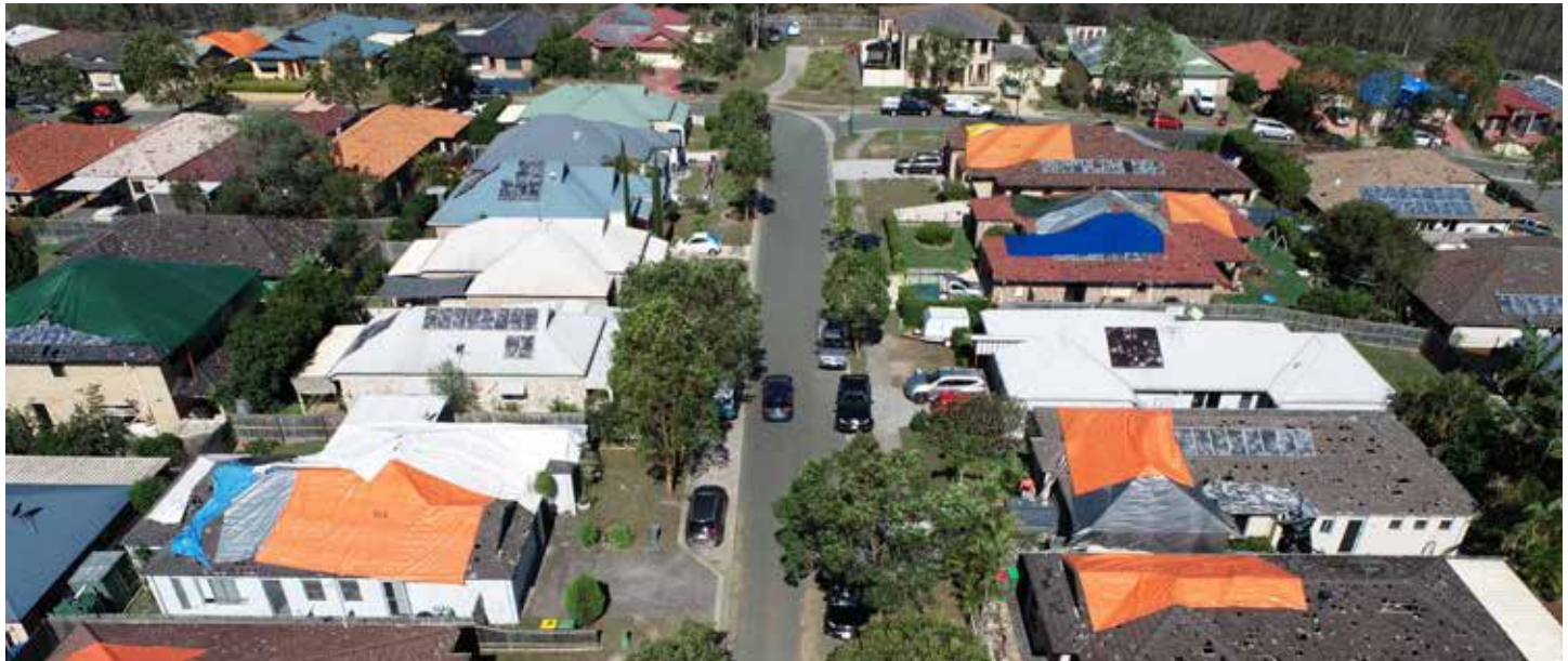
Tiled roofs were destroyed by the hailstones, with many needing to be fully replaced.
