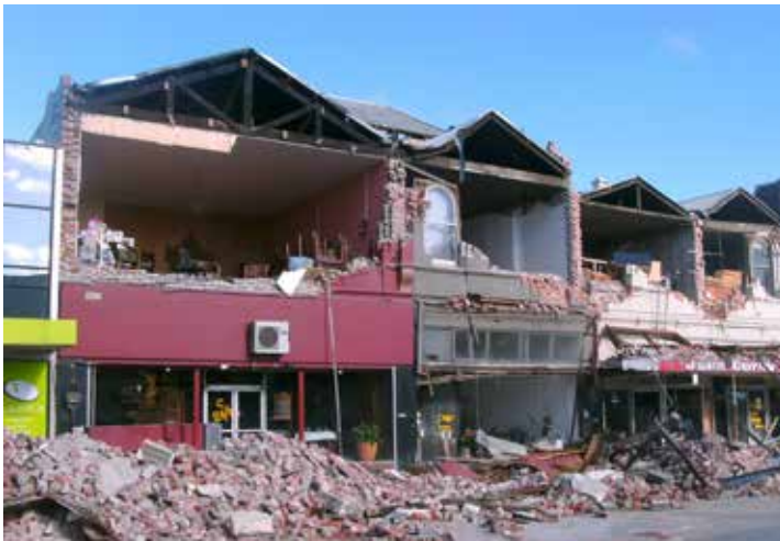
Silt and ground water were pushed to the surface, and an average of 70 aftershocks shook the ground each day.
