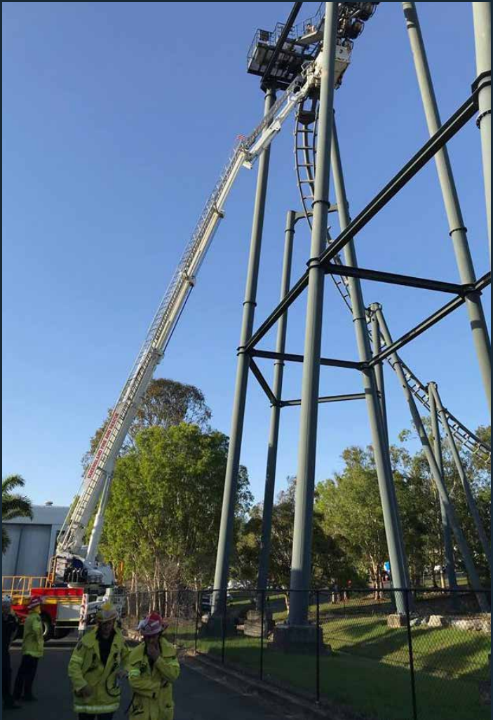
In February crews from C Shift Gold Coast North and Gold Coast South Commands attended an exercise at Movie World to test the theme park emergency response plans and the deployment of QFES specialist technical rescue and aerial resources. The exercise was successful with a hot debrief held post exercise.
