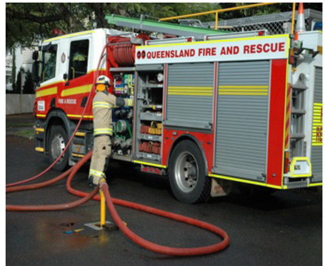
Figure 2 – Use of Hydrant System
