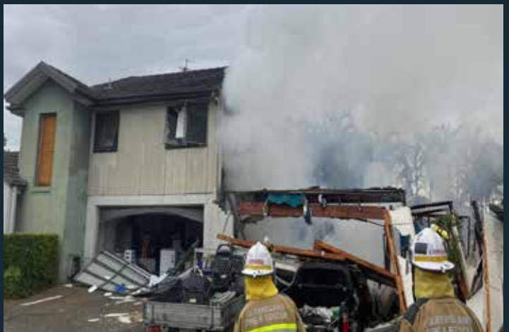
Fire and Rescue Service crews responded when a two-storey house was severely damaged by an explosion in Murrumba Downs.
