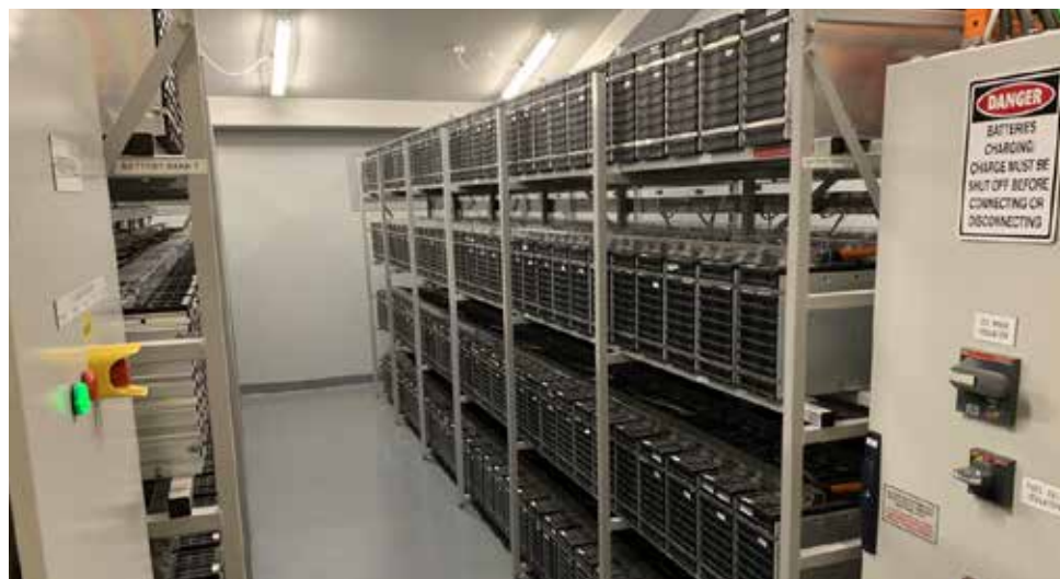
The explosion was caused by the batteries producing hydrogen gas as they decomposed.
