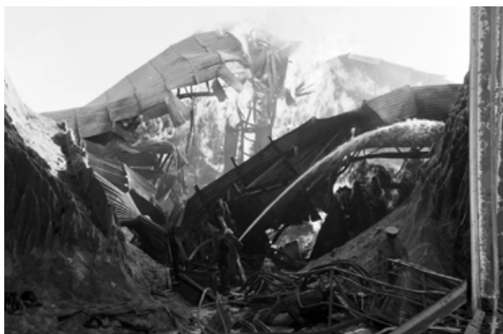
The mountain of sugar was 150 metres long, 45 metres wide and 27 metres high. Photo from Queensland State Archives.
