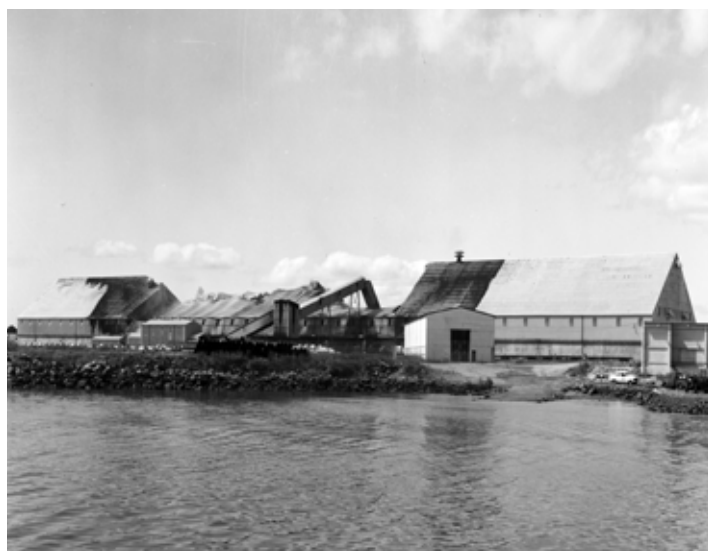
Built just four years earlier, the terminal was 300 metres long and could hold 10 per cent of Australia's annual sugar production. Photo from Queensland State Archives.
