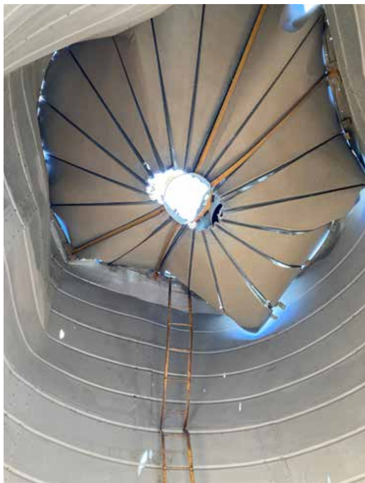
The silo's roof was on the verge of collapse during the rescue.
