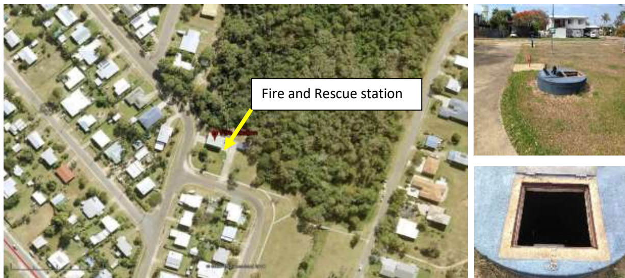
Figure NR 1 Forrest Beach Fire and Rescue station and surrounding suburban setting.
