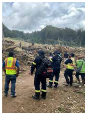
AUS-1 DART deployed to PNG to help local authorities respond to a landslide.
